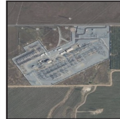
4. PG&E Bellota Substation
