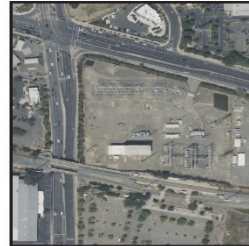
3. PG&E Brighton Substation
