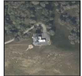
5. PG&E Clayton Hill Repeater Station
