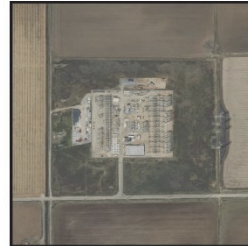
2. PG&E Rio Oso Substation
